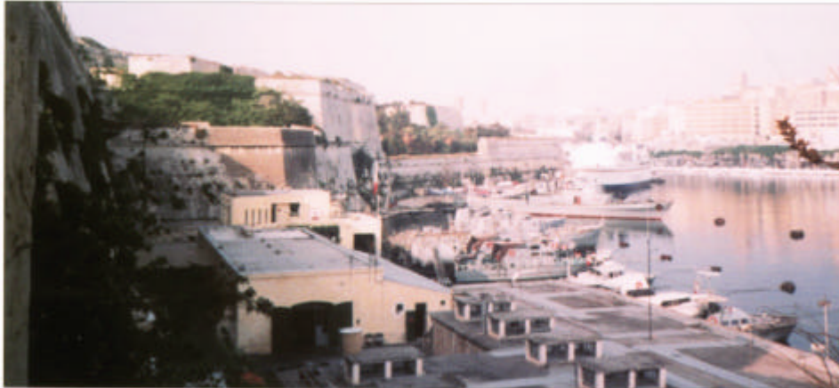
The harbour and bastions viewed from the far end of the Garden
